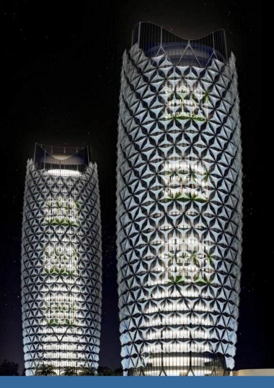
Twin Al Bahr Towers Abu Dhabi: the facade of this unique building react to the sun by closing and opening
